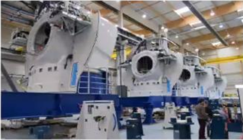
Turbines assembly – Saint-Nazaire – General Electric
