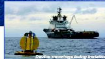
Device moorings being installed
