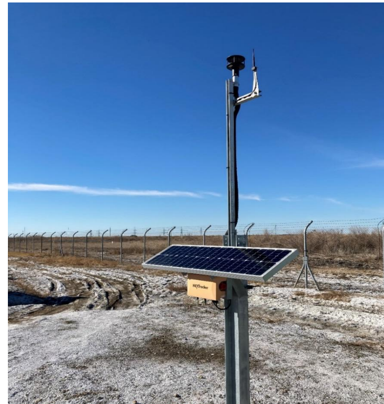
Wind speed measurement Trackers go to stow at 11 m/s. Structure designed for 47 m/s to 51 m/s
