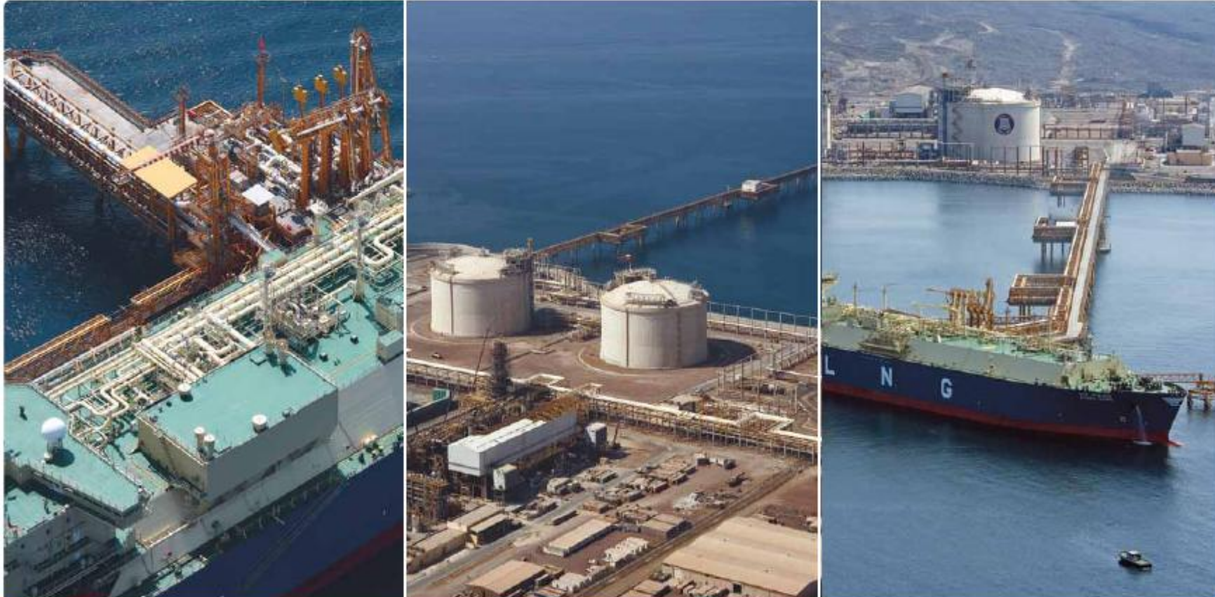
The Yemen LNG liquefaction complex in which Total is the main shareholder. Construction of the site mobilized 10,000 people.
