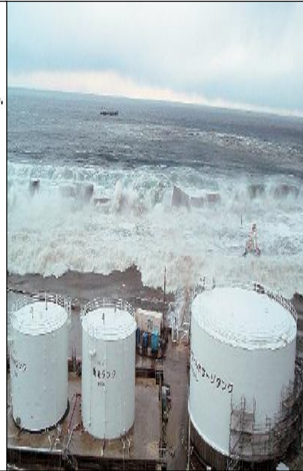
Tsunami wave overrunning the sea walls and flooding the Fukushima Daiichi nuclear power plant on 11 March 2011 (photo taken from unit 5).
